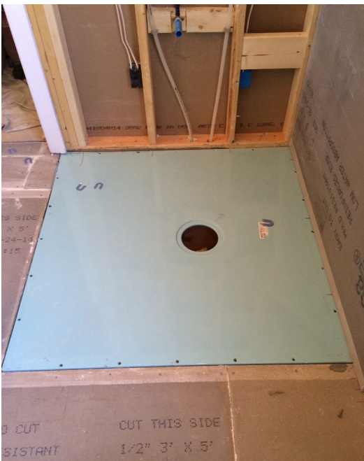
Classic shower base installed on joists.
